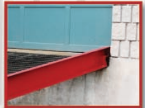
PICTURE SHOWING apron at top of ramp with 8.5 degree bend.
